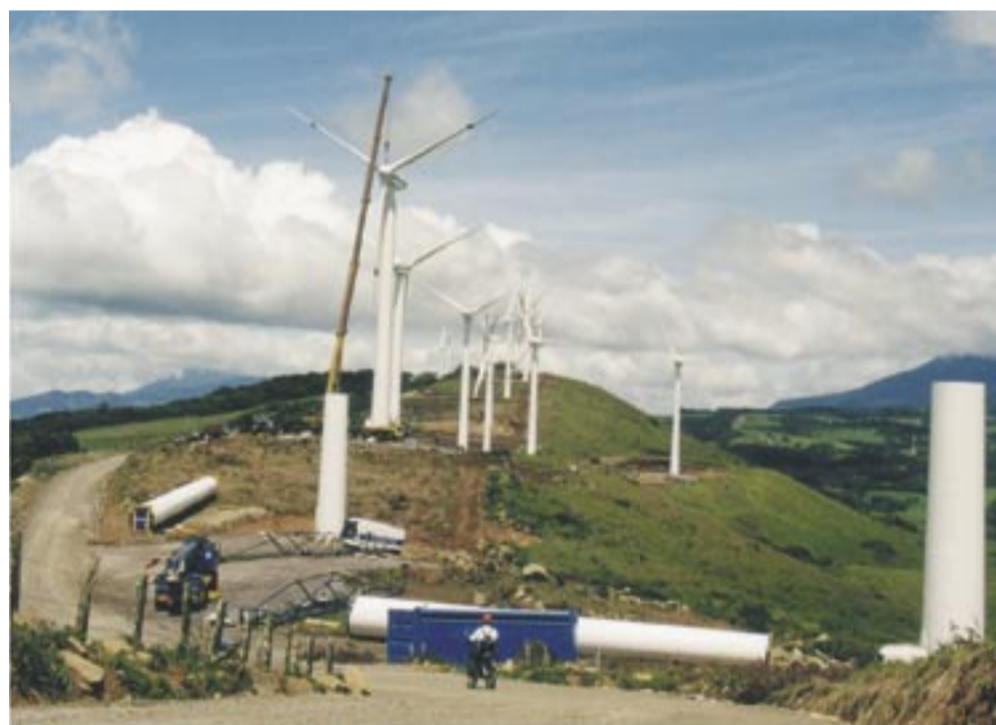
ECN was responsible for training, farm lay out, environmental impact assessment and grid feed in study of the 20 MW wind farm at Tejoina, Costa Rica.
