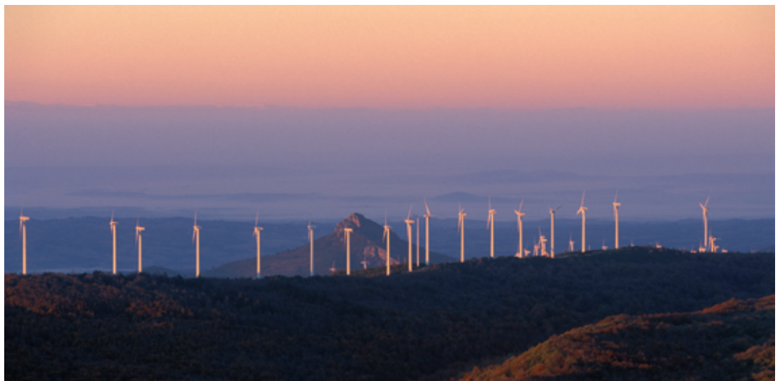
Figure 1: 33 MW Alaitz Wind Farm.
