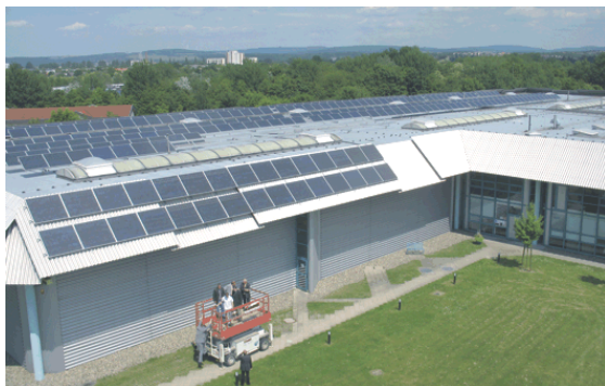
Figure 1: Industrial site of Hübner GmbH in Kassel with the 104 kWp PV generator
